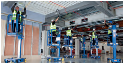
Power Tower's Pecolift in use for the 'fit-out' of the News International offices in Central London, UK.
